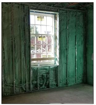
The masonry walls of the existing building are insulated with 2 1/2 inches of spray foam insulation inside the original structure. In the new addition, the rain screen walls include 3  $\frac{1}{2}$  inches of mineral wool insulation over 2  $\frac{1}{2}$  inches of spray foam which will reduce thermal bridging which significantly impacts building envelope performance.
