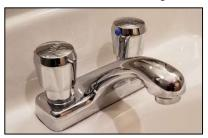
The building utilizes high efficiency fixtures to reduce potable water consumption. Grossman Hall is equipped with low flush toilets and 1/8 gallon-per-flush urinals. The project achieves a 45.5% water use reduction though the use of the very high efficiency water fixtures.
